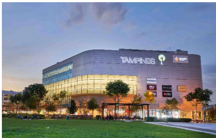
Tampines 1 building, which has obtained BCA Green Mark GoldPlus Certification. Image credit: FCT
